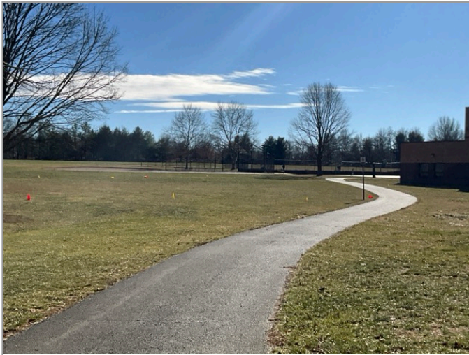
ACCESSIBLE ROUTE TO PLAYGROUND
