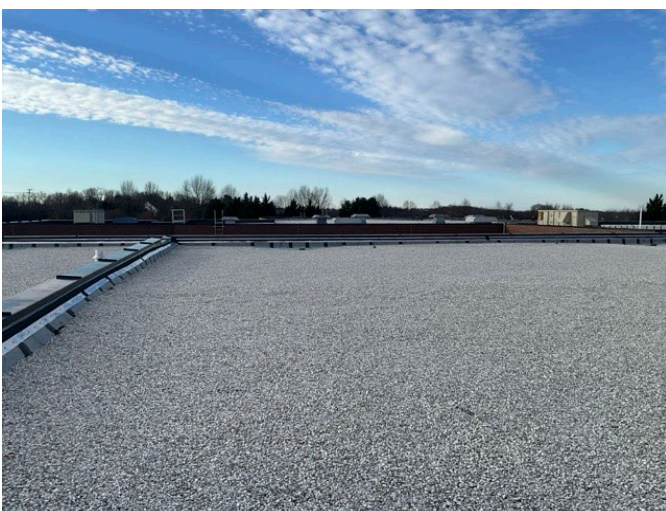
5 - PRIMARY ROOF OVERVIEW
