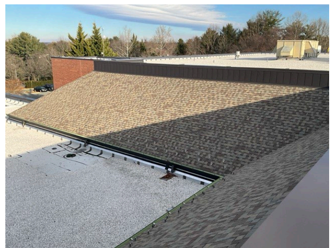
6 - SECONDARY ROOF OVERVIEW
