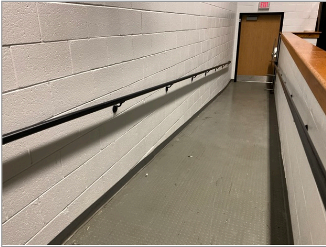
ACCESSIBLE INTERIOR RAMP
