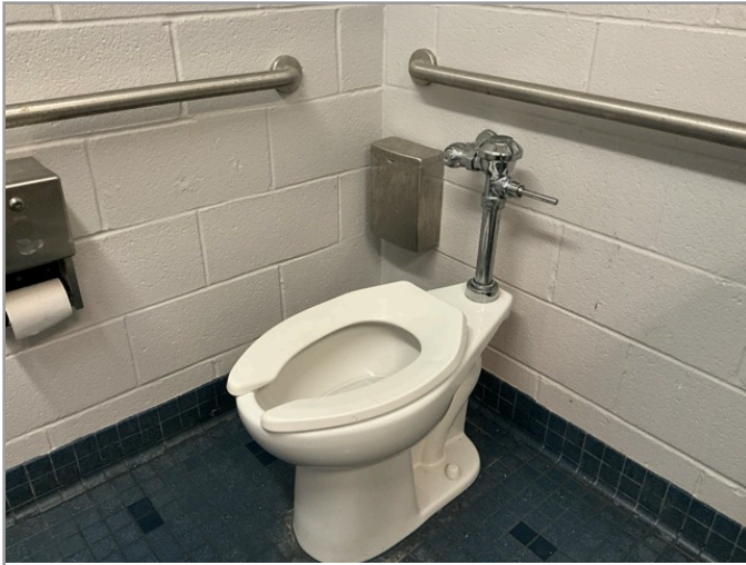
TOILET STALL OVERVIEW
